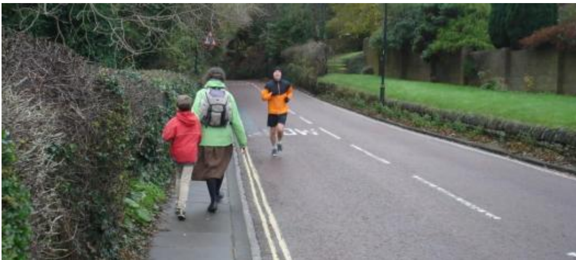
Narrow pavement on Margery Lane, on only one side of the road. Observe the 'slow' markings for motorists: most of them do not.
