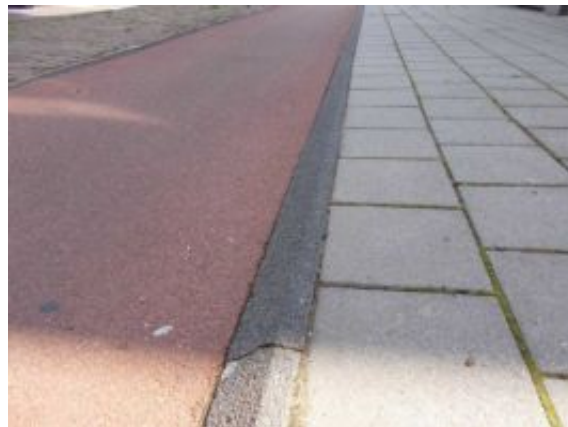
30° splay kerb from The joy of kerbs by City Infinity, p. 31
